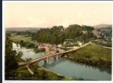
[Dinham Bridge and Ludlow, England]
