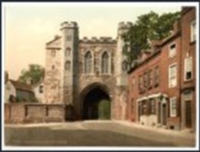
[ Edgar Tower, Worcester, England ]
