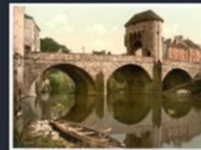
[ Bridge over the Monnow, Monmouth, England ]
