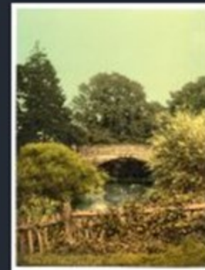
[ Penshurst Bridge, Tunbridge Wells, England ]
