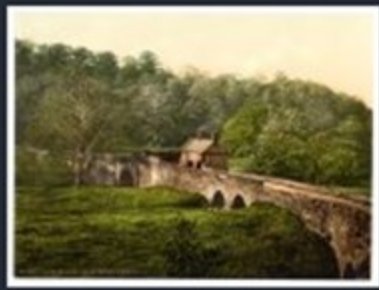
[Ambergate, Halfpenny Bridge, Derbyshire, England]
