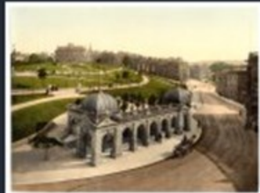
[Buxton, pump room, Derbyshire, England]
