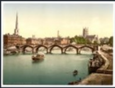
[ Severn Bridge, Worcester, England ]
