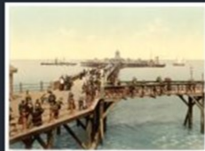
[ The jetty, I., Margate, England ]
