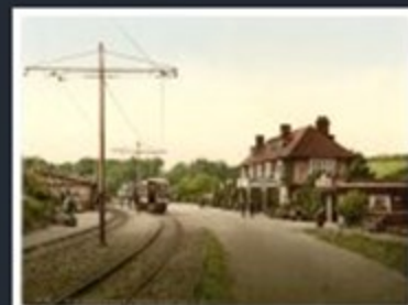
[ Groudle Glen Hotel and tram station, Isle of Man, England ]
