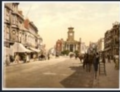
[ South Street, Worthing, England ]
