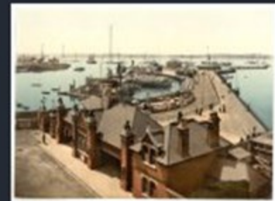
[The pier, Southampton, England]
