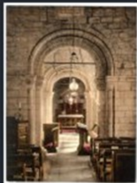
[Studland Church, interior, Swanage, England]
