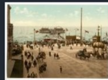
[The North Pier, Blackpool, England]
