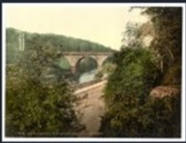
[Ambergate, railway bridge over River Derwent, Derbyshire, England]
