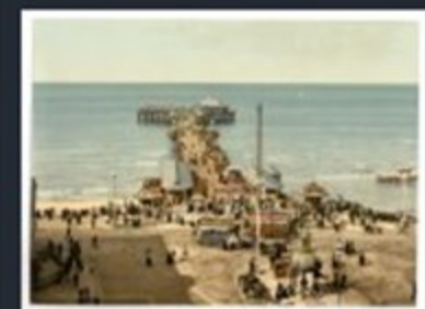
[The North Pier, Blackpool, England]
