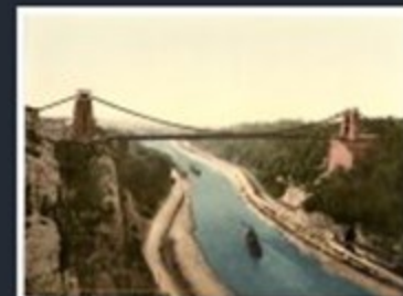
[Clifton suspension bridge from the north cliffs, Bristol, England]
