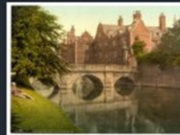
[St. John's Bridge from the grounds, Cambridge, England]
