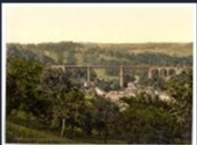
[Viaduct, I., Lydbrook (Lower), England]
