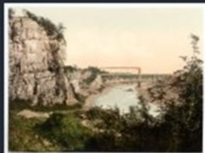
[Tubular Bridge, Chepstow, Wales]
