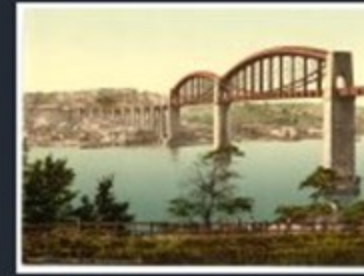
[ Saltash Bridge, Plymouth, England ]
