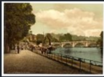
[ Richmond, the bridge, London and suburbs, England ]
